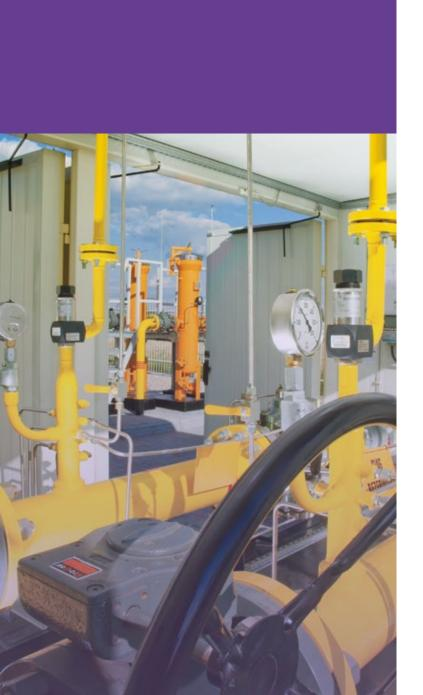
monitor the operation of the PRMS station remotely, in real-time
